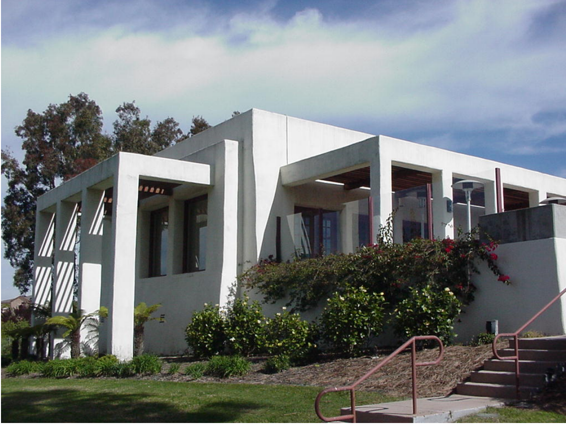
Reception Room Addition
